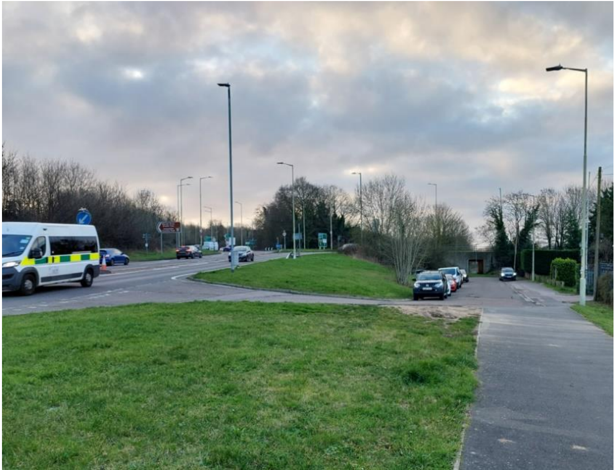
Figure 1 – Level Difference at Site Access Location
